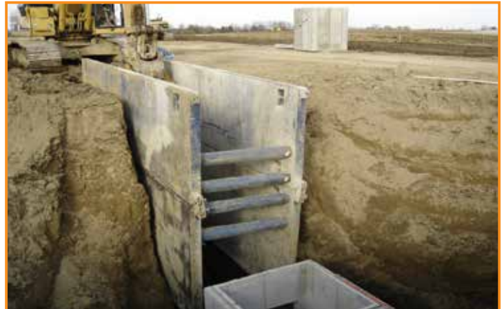
Stacked Trench Shields
