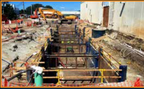
Slide Rail Shoring
