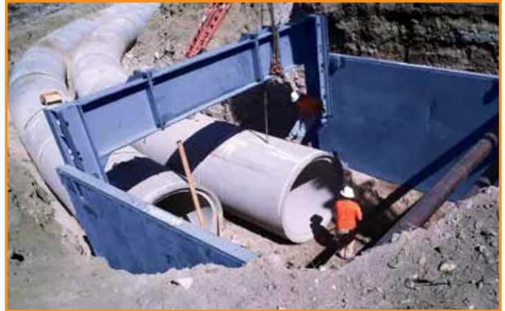
A 6M Series Trench Shield with Height Adapters
